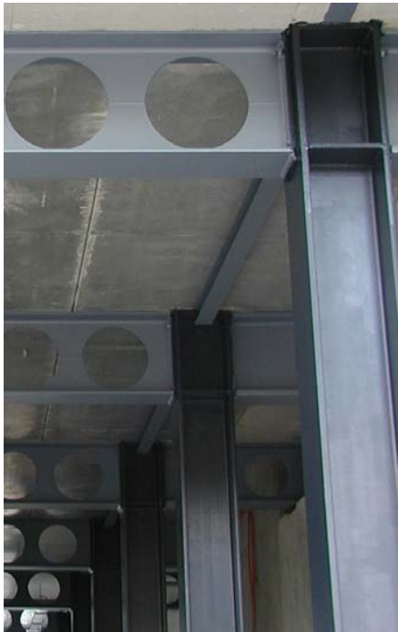
Figure 16: Beam to column connection
